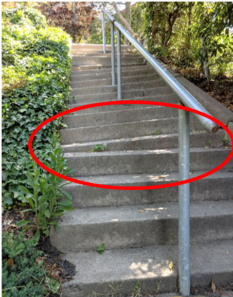
Uneven/ broken steps on concrete path
