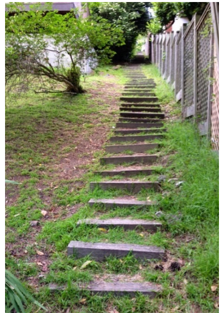
Steep path, no handrails
